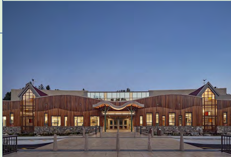
The new Sandy Hook school building that utilizes CPTED. Note the see-through fence to limit hidden areas, and the large glass windows for increased surveillance of the area.
